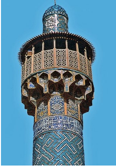
Minaret of Shah Mosque, Isfahan, Iran, 1611-38
